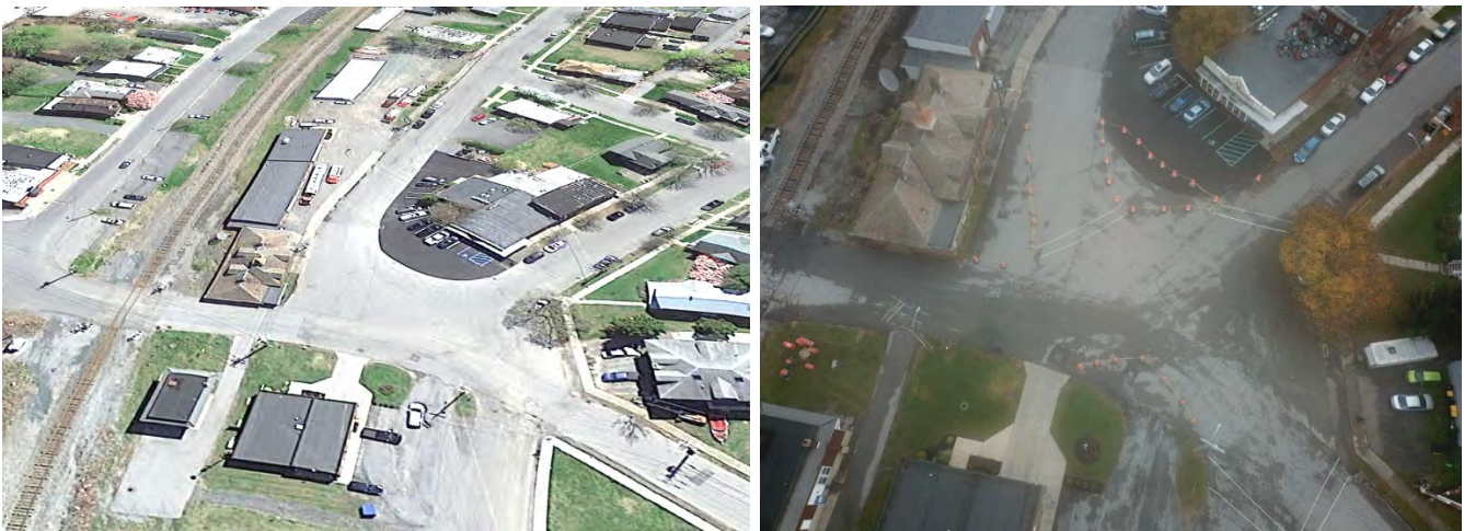
Figure 2. Depot Square Demonstration Project (Before/During)
