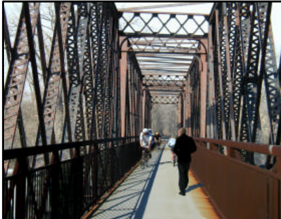
Figure 4b: Delaware Avenue Bridge After.
