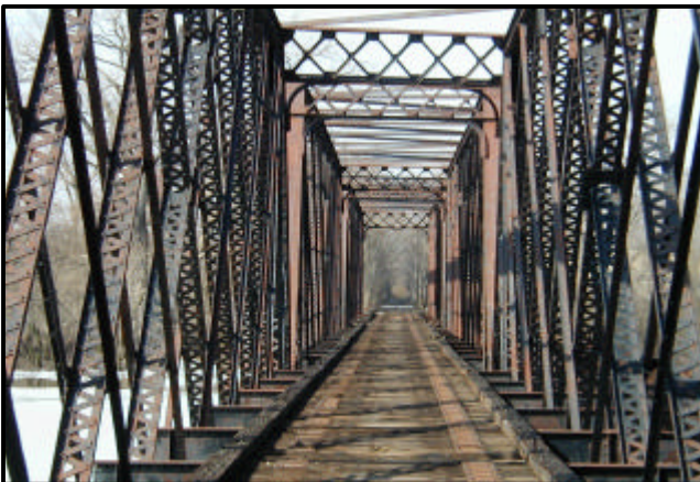
Figure 4a: Delaware Avenue Bridge Before.
