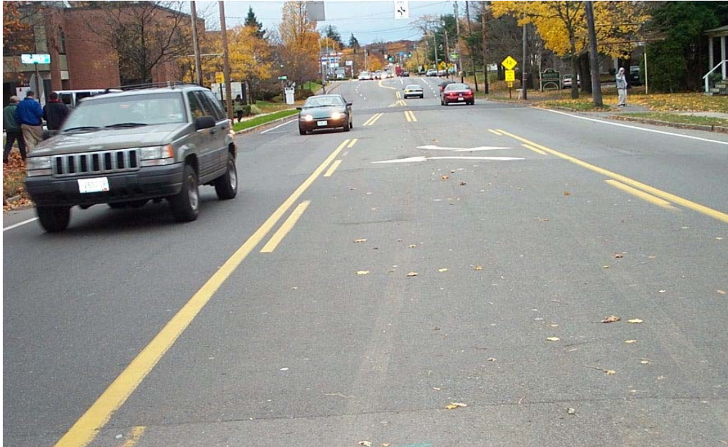
Road Diet, Portland ME A four-lane undivided roadway (in background) was restriped as a three-lane road with a flush turn lane (in foreground).
