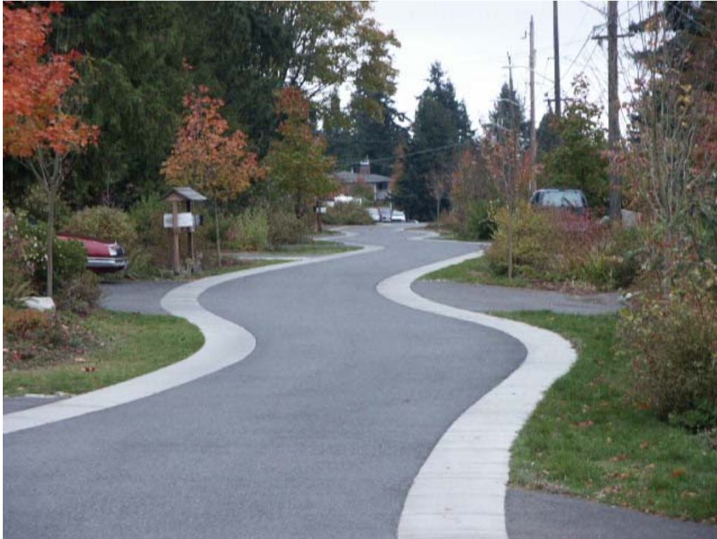
Traffic Calming Project with Serpentine Street in Washington
