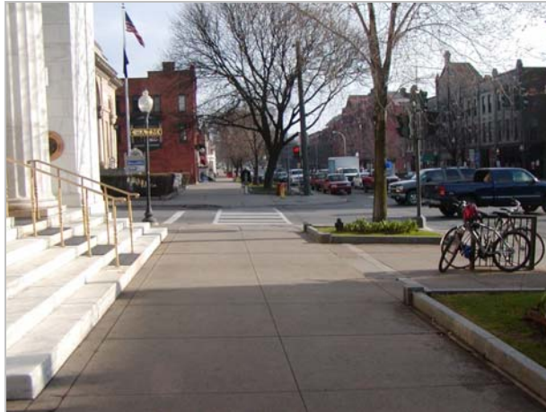
A view of bicycle and pedestrian facilities on Broadway (2005) in the City of Saratoga Springs, New York.
