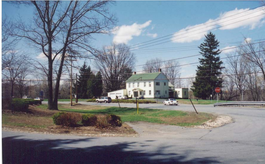
Existing conditions (2003) of the Gilbert Road and Lake Avenue intersection in the City of Saratoga Springs, New York.
