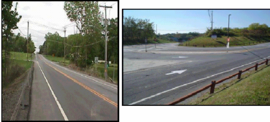
Existing conditions (2004) in the Route 151 corridor in the Town of East Greenbush, New York.
