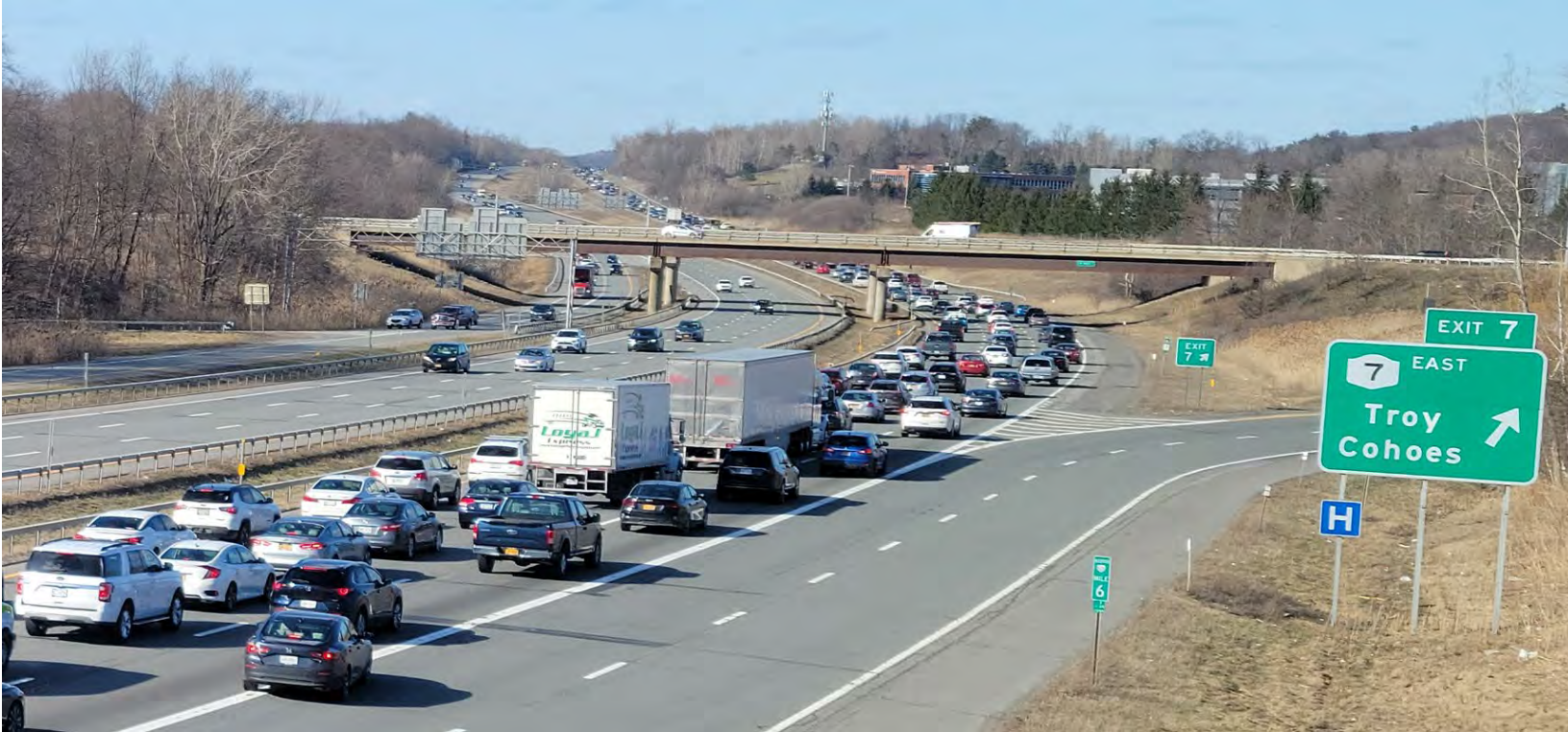
Above: traffic congestion on I-87 near Exit 7. Per-mile emission rates of slow-moving vehicles can be up to four times greater than vehicles moving at free flow speeds. Photo courtesy of Creighton Manning Engineering.
