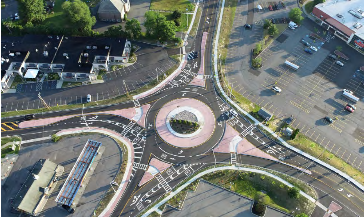
Above: roundabout on Route 9W in Glenmont. Photo courtesy of Creighton Manning Engineering.
