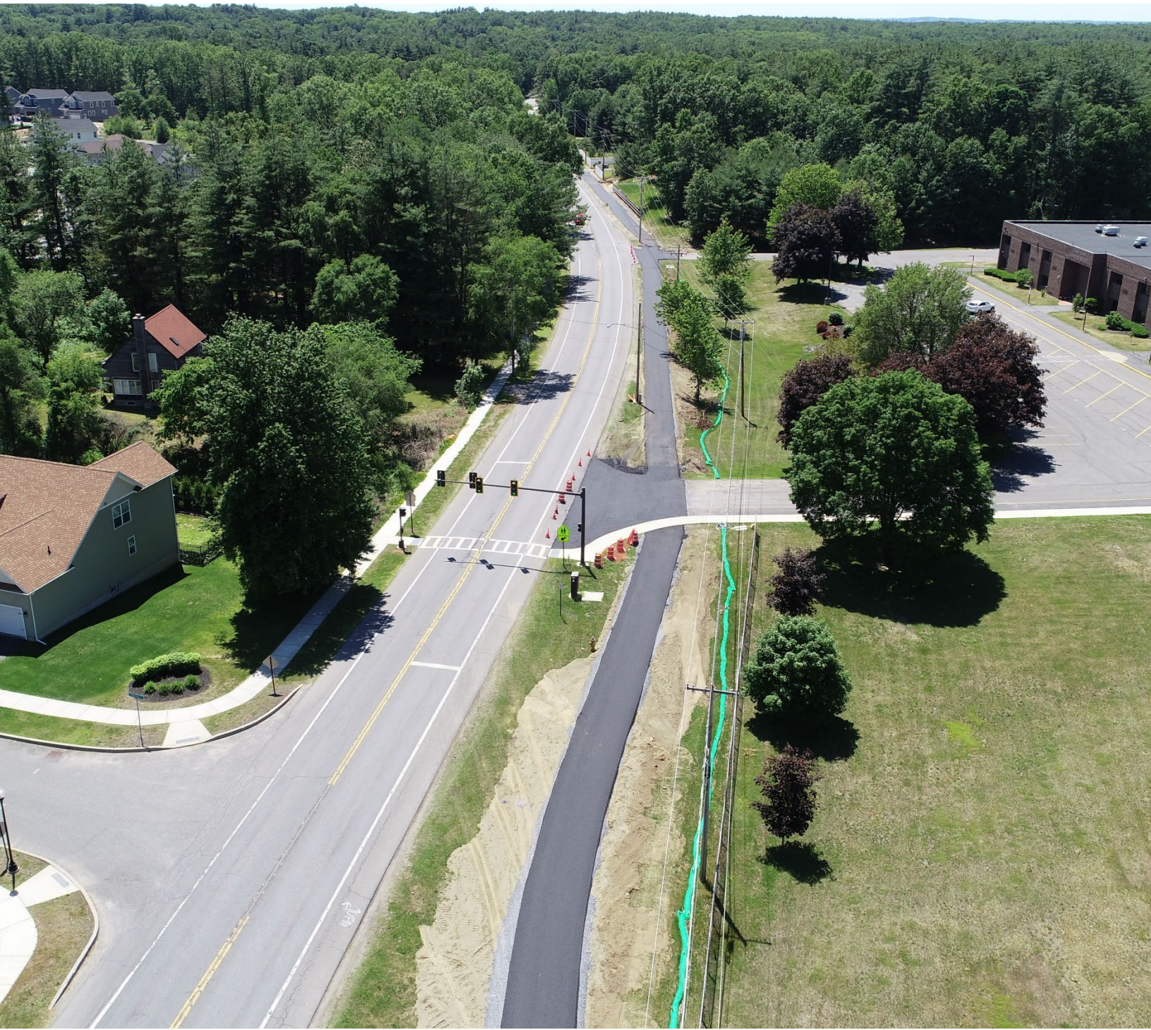
Above: Geyser Road Trail in Saratoga Springs. Photo Courtesy of GPI.
