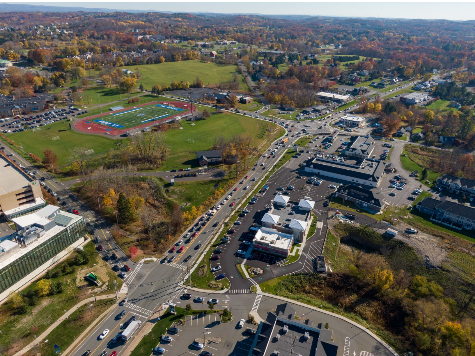
Above: traffic on US-4 in Troy and North Greenbush, near Hudson Valley Community College. Photo courtesy of WSP.
