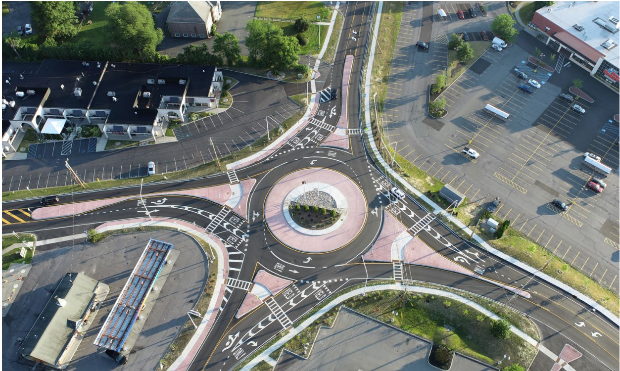
Above: roundabout on Route 9W in Glenmont. Photo courtesy of Creighton Manning Engineering.
