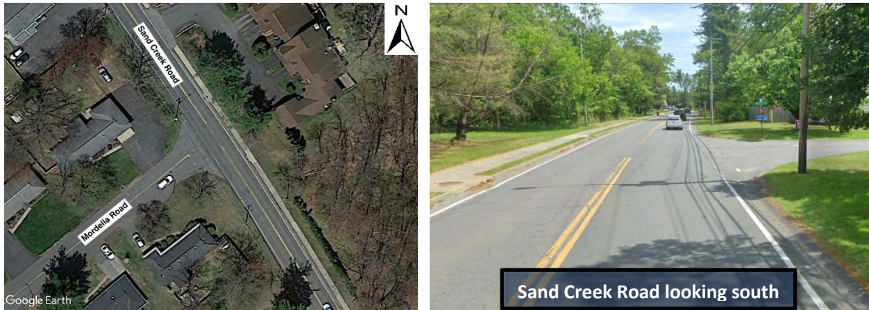
Figure 2.10: Sand Creek Road and Mordella Road Intersection
